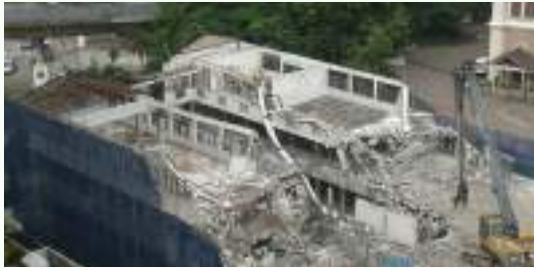
拆除B栋三层旧校舍
